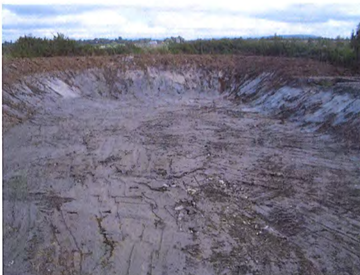
Cleaning of the inlet lagoon has been complete
