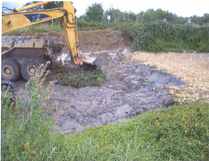
Cleaning and removal of silt and vegetation from the inlet lagoon
